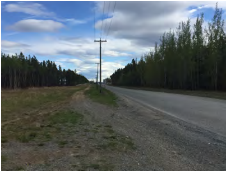
Range Road at C-15B (facing S)
