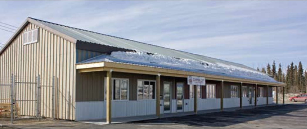
The new offices of Canyon City Construction are on the corner of Tlingit and Platinum. The KDFN company is a for-profit business that employs qualified citizens whenever possible.
