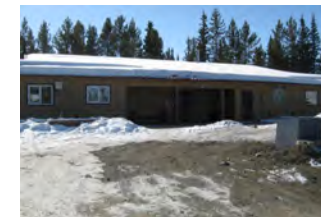
Kenädän Ku House of Learning building at 5 O'Brien Place
