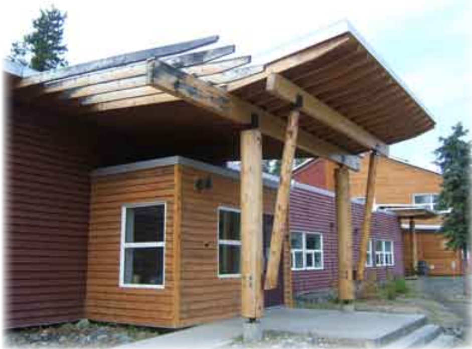
Community Services helps to keep Kwanlin Dün buildings like our Health Centre in shape by doing repairs, renovating office space when needed and general upkeep.
