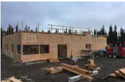
The Multi-purpose Gymnasium is quickly taking shape.
